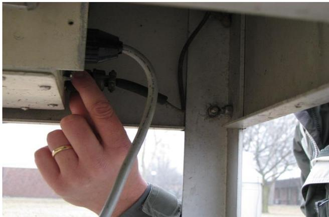
2. Unscrew the four screws securing the sensor to the frame of the collector. Be careful not to drop or misplace the screws as they will be re-used with the replacement sensor.
