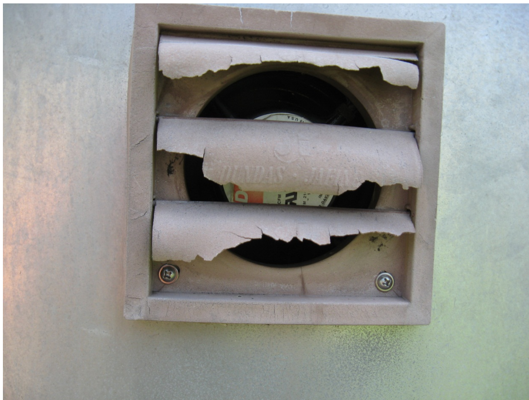
Figure 5-4. – ACM MDN Cooling Fan Louver
