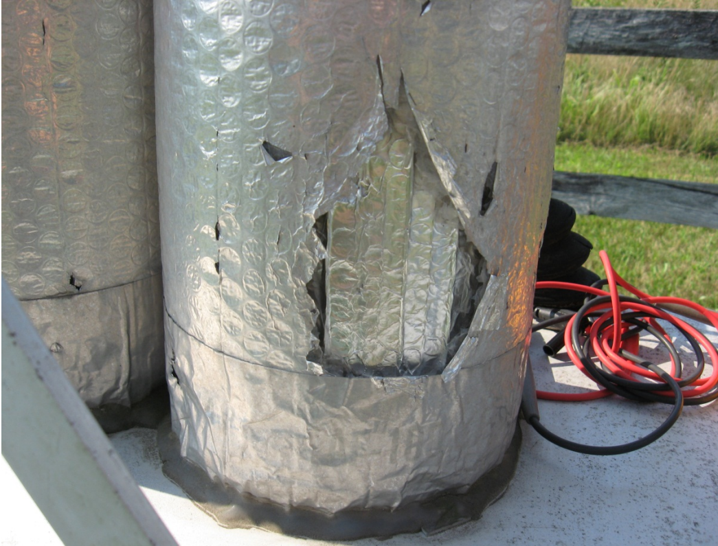
Figure 5-1. – ACM MDN Chimney Insulation
