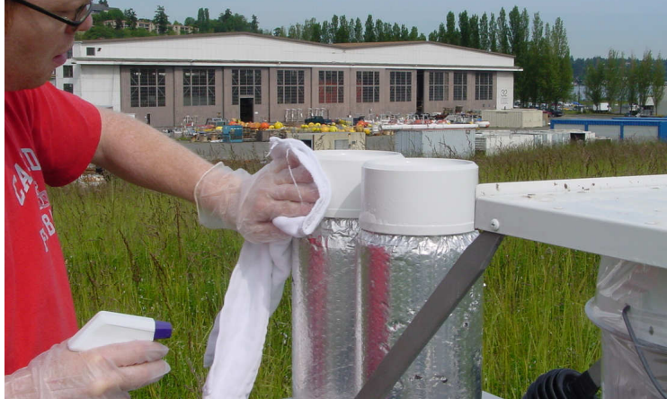
Wiping down chimneys.
