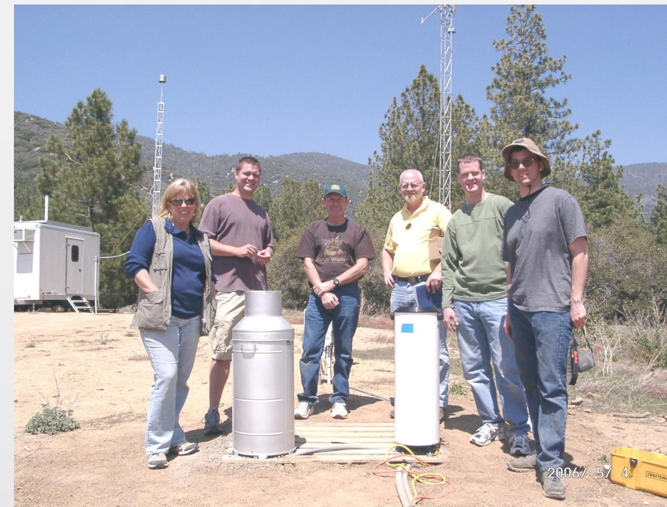
April 2006 NOAH IV installed at CA94
